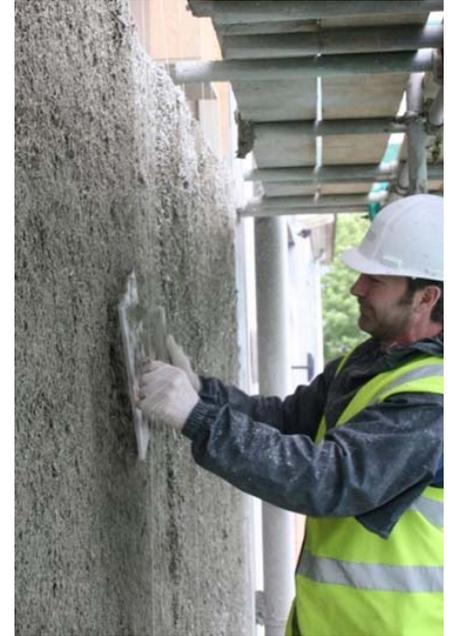
A final remarkable characteristic is that lime-hemp walls retain heat longer due to their specific heat capacity, so they can have some of the thermal characteristics of insulation and some of the thermal mass characteristics of heavy mass materials, like concrete. This was seen to good effect in a BRE study of the Haverhill lime-hemp houses in Sussex.
